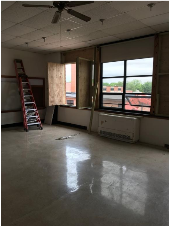
Temporary opening for material
